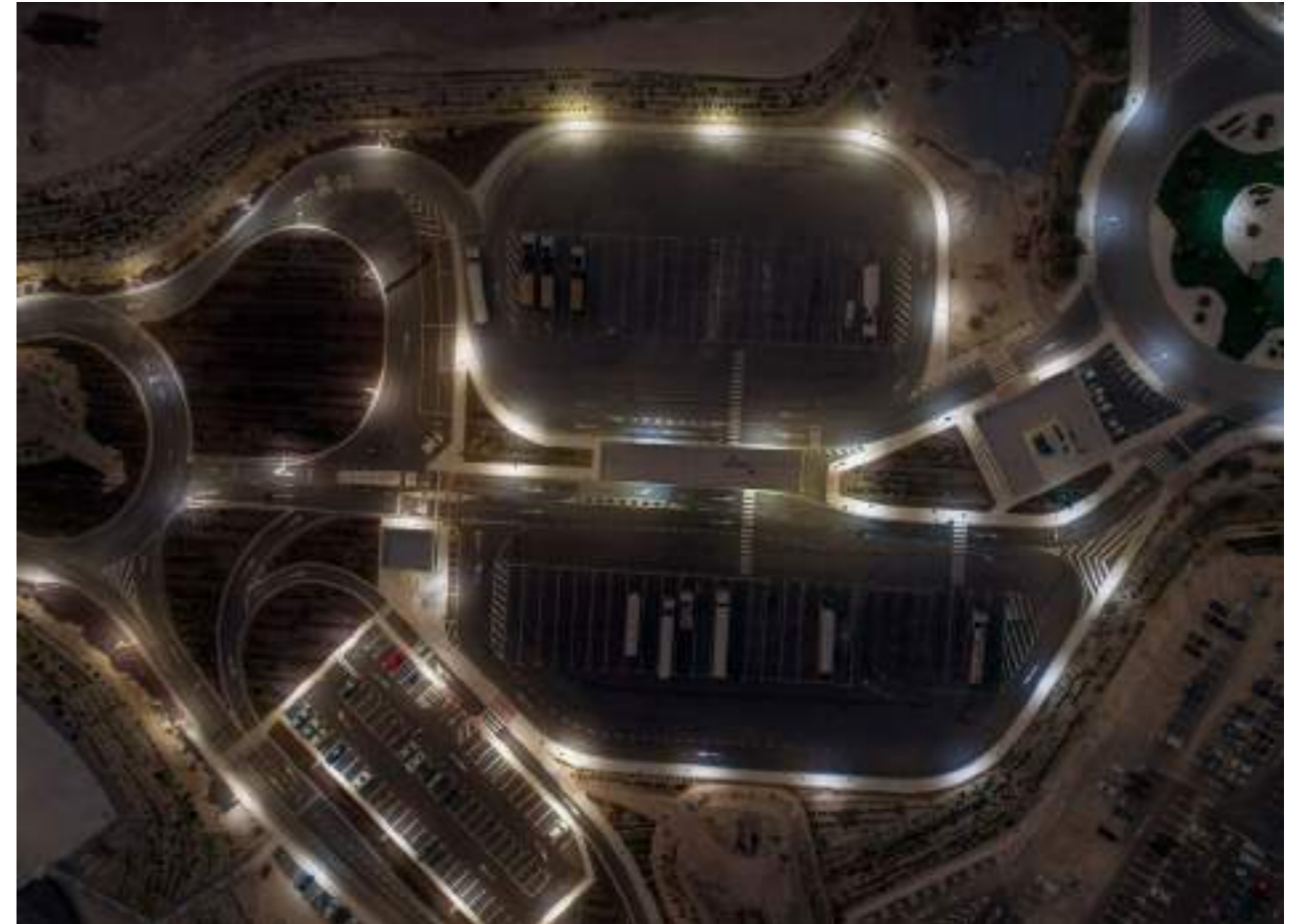
→ LED lighting throughout the Cosentino industrial park
